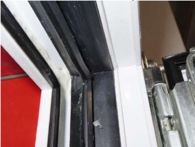
Picture 15 Central rebate seal at top
