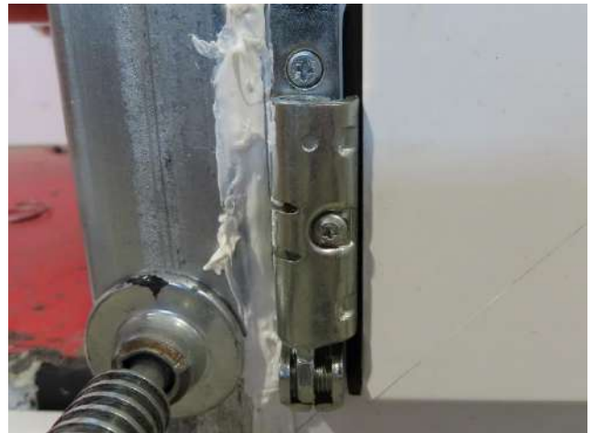
Picture 6 Hinge view of opening side, inactive casement at bottom
