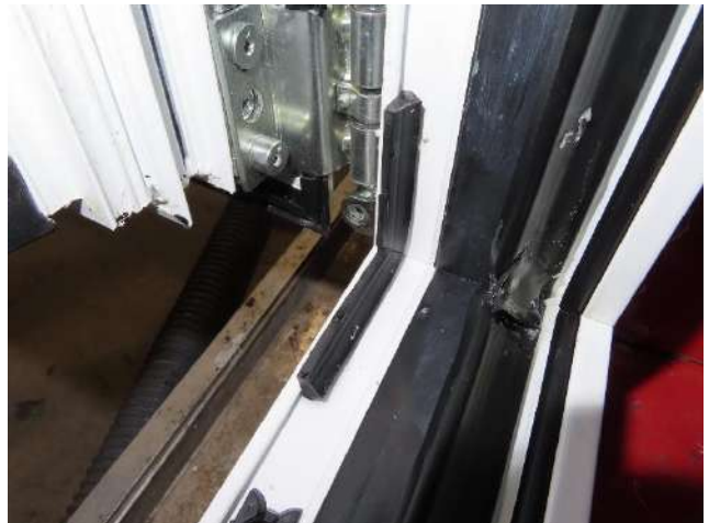
Picture 34 Additional sealing plane at corners
