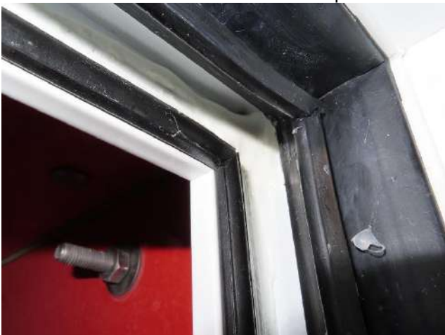
Picture 17 External rebate seal at top
