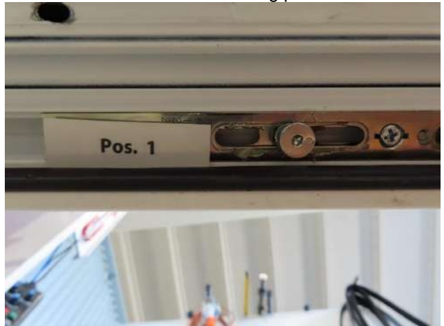
Picture 36 Locking situation 1, casement
