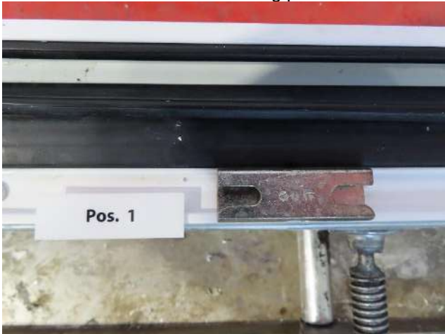
Picture 35 Locking situation 1, frame
