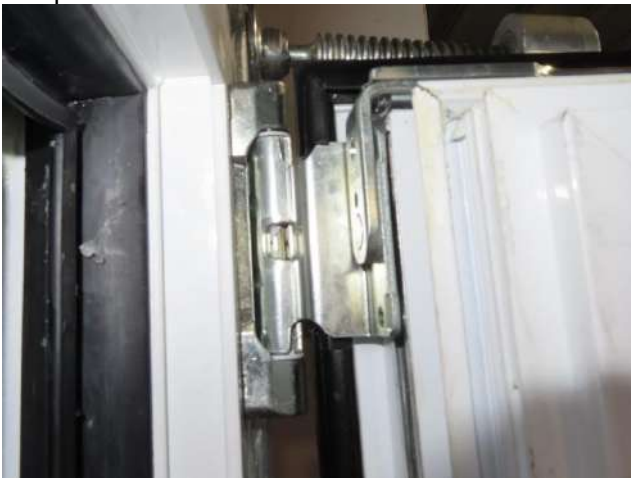
Picture 11 Hinge rebate view, active casement at top
