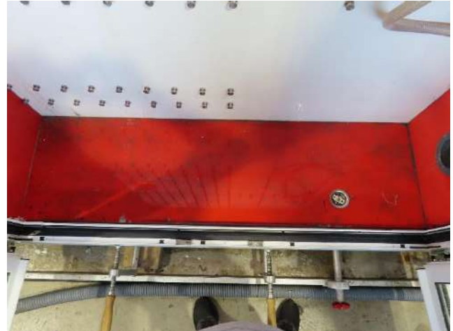
Picture 28 Frame at bottom with rebate drainage slot
