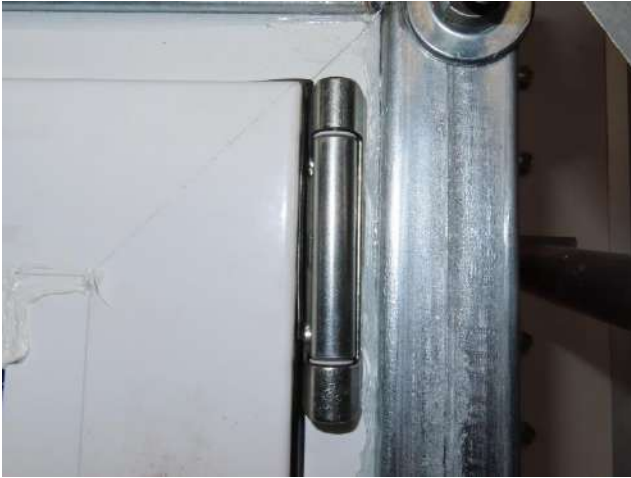
Picture 7 Hinge view of opening side, active casement at top
