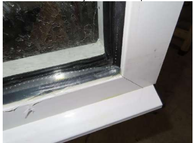
Picture 24 External glazing gasket and additional sealing
