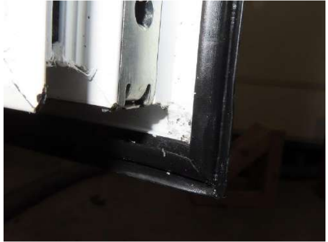
Picture 14 Casement seal at bottom
