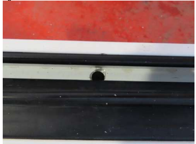
Picture 30 Drainage drilling
