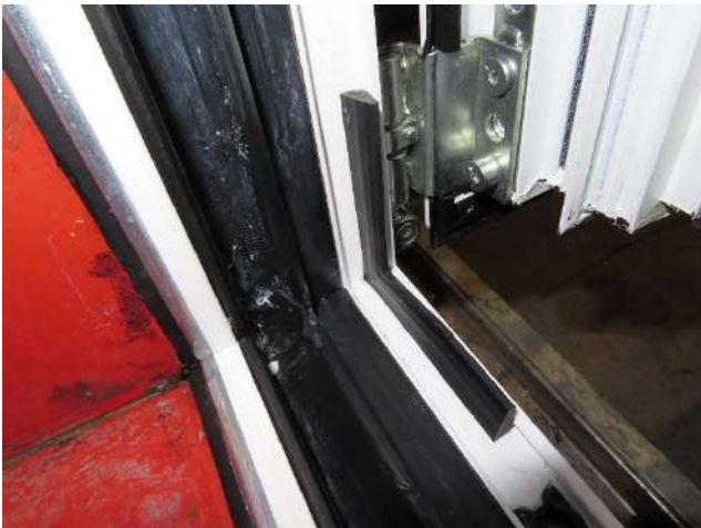
Picture 33 Additional sealing plane at corners
