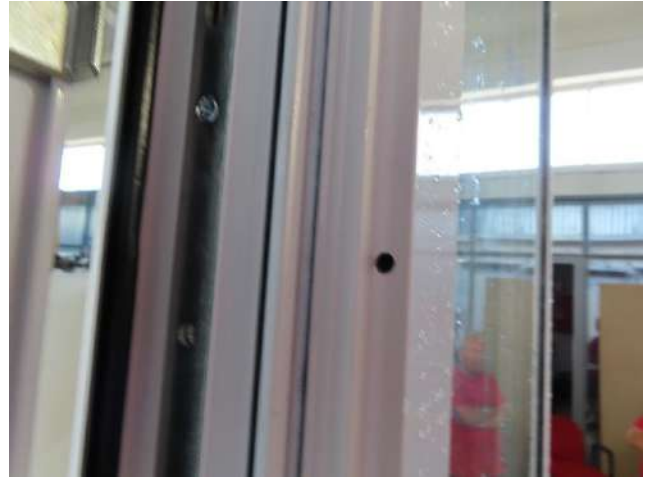
Picture 26 Vapour pressure equalisation drills, casement lateral
