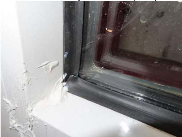
Picture 23 Internal glazing gasket
