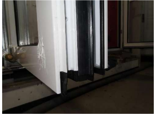
Picture 20 Dummy mullion at bottom
