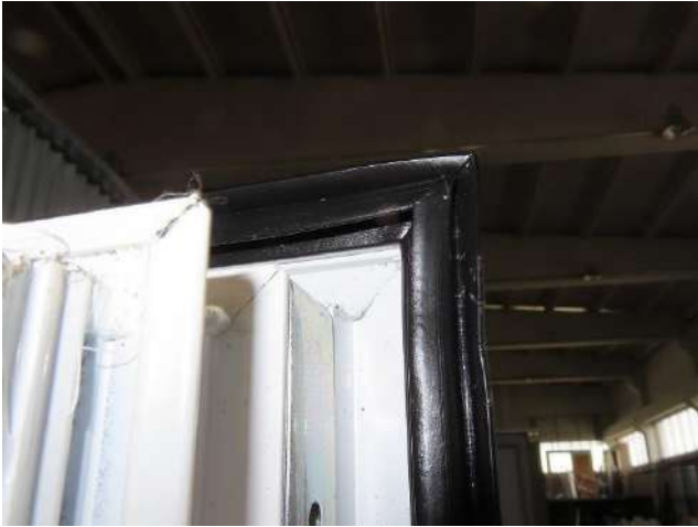
Picture 13 Casement seal at top
