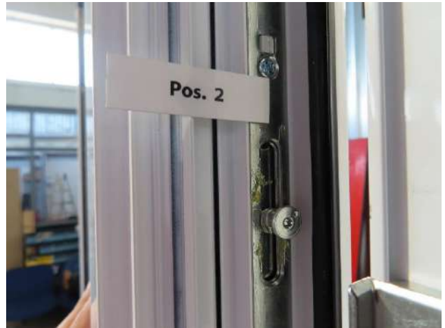
Picture 38 Locking situation 2, casement
