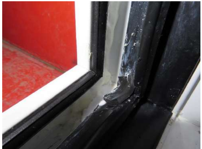
Picture 18 External rebate seal at bottom
