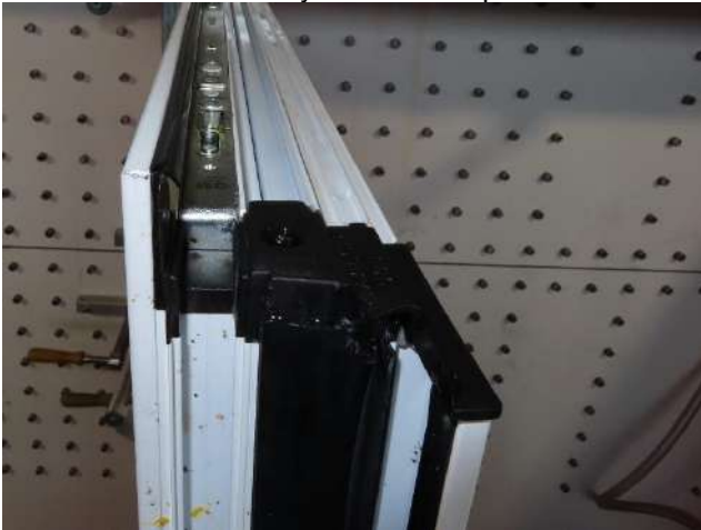
Picture 21 Dummy mullion end cap at top
