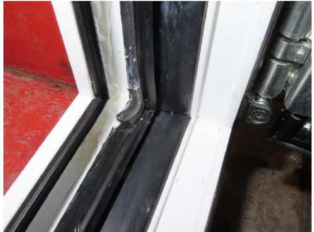
Picture 16 Central rebate seal at bottom
