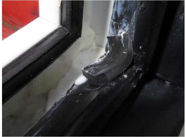
Picture 32 Corner design of central gasket
