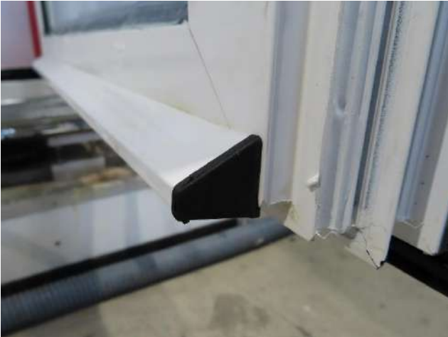
Picture 27 Weather bar, casement
