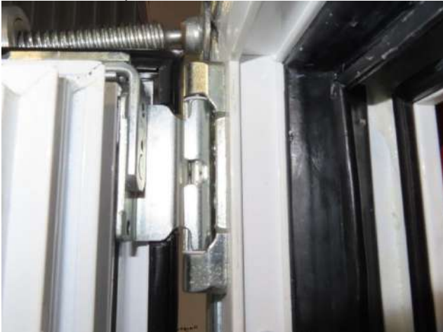
Picture 9 Hinge rebate view, inactive casement at top
